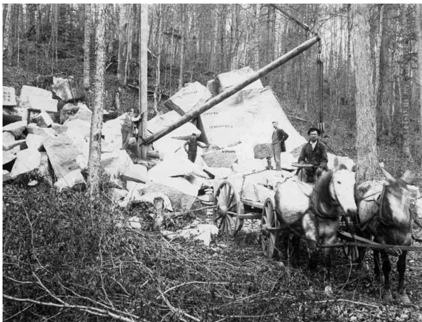
Figure 33. Granite teamster at a Woodbury, Vermont, quarry. Note the brake wheel.
