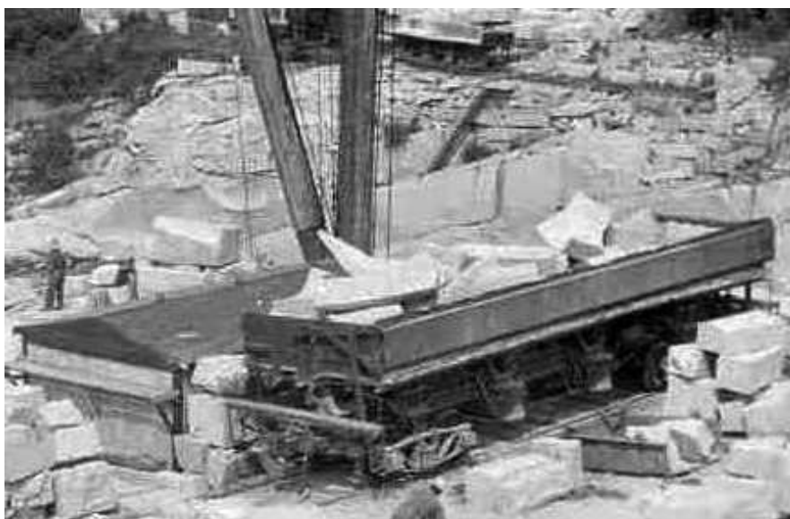
Figure 25. Side-dump grout car.
