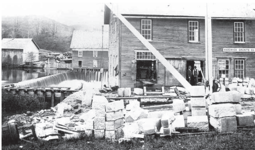
Figure 35. Dam at the Hardwick Granite Co. polishing mill, Hardwick, Vermont. A turbine in the basement powered gate-type and vertical polishing machines on the main floor.
