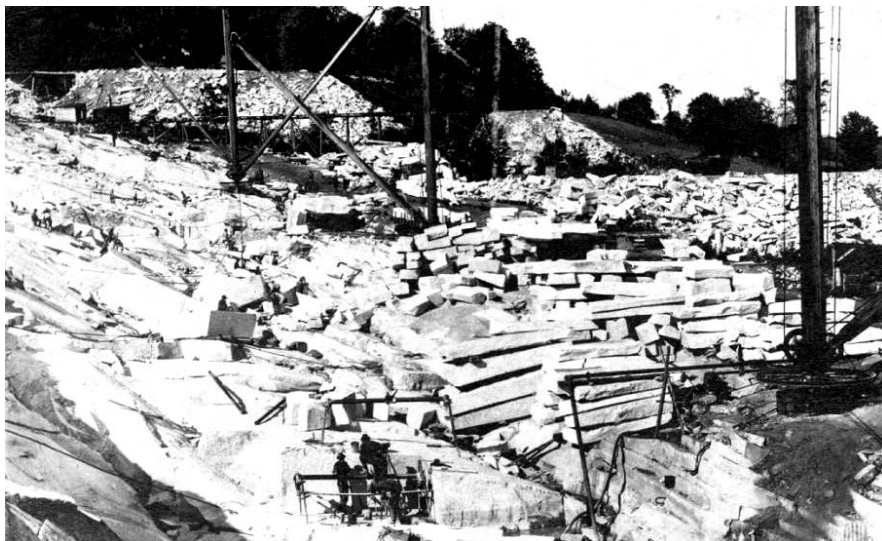
Figure 23. Woodbury Granite Co. White Quarry in Bethel, Vermont, with grout trestles in the background. Three grout piles are visible.
