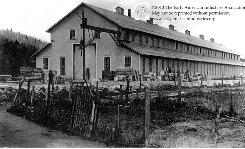
Figure 3. Shed No. 1, the main shed of the Woodbury Granite Co., Hardwick, Vermont, ca. 1905-10, an example of a straight shed. The upper level with clerestory windows had the height to accommodate two overhead traveling cranes—one forty-ton and one twenty-ton.
