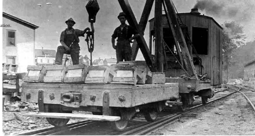
Figure 19. Coal-fired locomotive crane shown loading and moving a transfer car. This locomotive crane acted as a switcher on the Woodbury Granite Co. (Hardwick, Vermont) railroad spur network. The lumber is on the left and the worker on the right is probably the crane operator.
