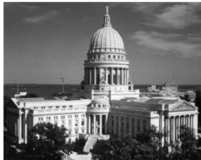
Figure 11 (below, left). State House, Harrisburg, Pennsylvania. Built in 1905 from Woodbury, Vermont, gray granite.
