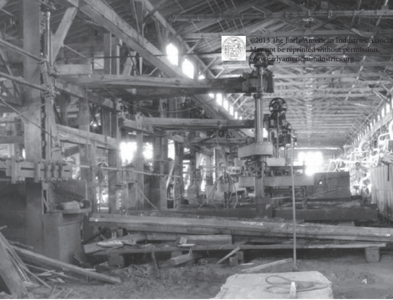
Figure 11 (left). A row of four boring machines at Jones Brothers Co., Barre, Vermont. Not visible are the pits beneath the machines needed to accommodate long columns.
