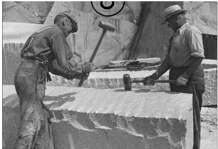
Figure 22. Trimming a quarry block with bull set and striking hammer.
