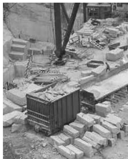
Figure 24. End-dump grout car.
