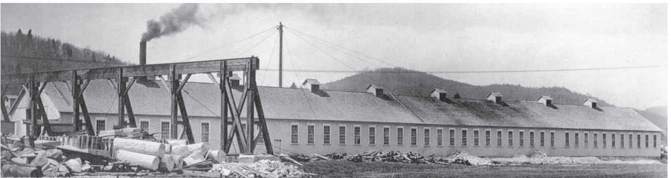
Figure 46 (below). Granite shed with string of eight ventilating cupolas.
