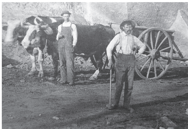
Figure 33. Ox cart and team at a Woodbury, Vermont, granite quarry. Before the railroad, carts were used to haul out waste granite.
