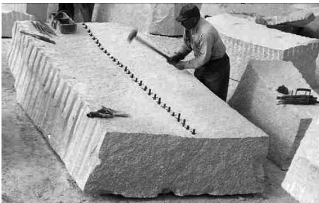
Figure 36. Driving the wedges.
