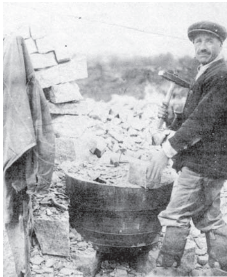
Figure 19 (left). Paving-block cutter using a reel hammer to trim a paving block over his chipping tub at the Rockport Granite Co, Rockport, Massachusetts.
