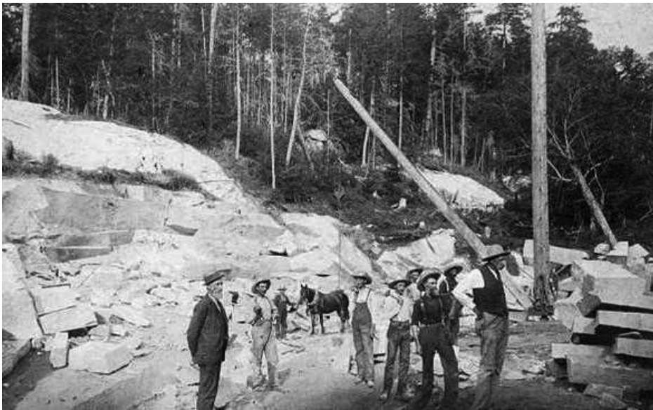
Figure 13 (left). Hillside quarry, Woodbury, Vermont, circa 1890s. Note the small dead-boom derrick and the horse, probably to power the derrick.
