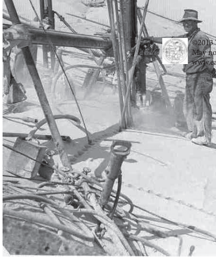
Figure 37 (left). A maze of compressed air hoses at a Barre, Vermont, granite quarry with a pneumatic quarry drill in the background.
