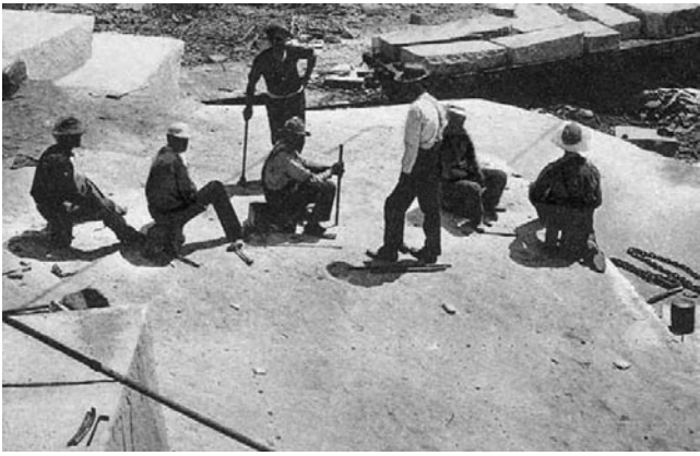
Figure 20. Double jacking deep holes.
