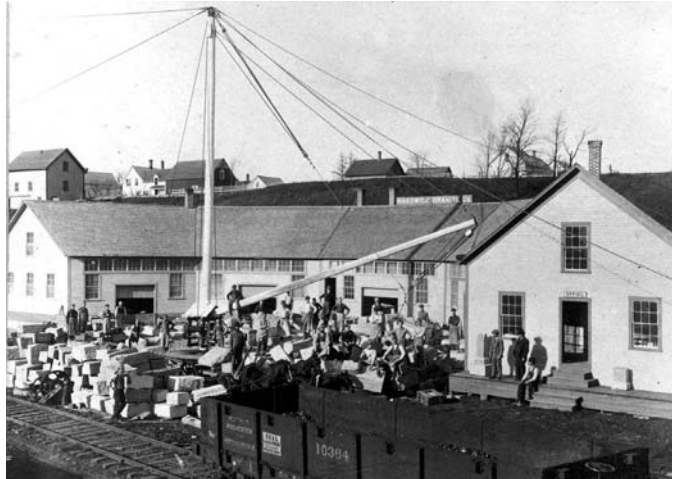
Figure 2. Horseshoe shed of the Hardwick Granite Co., Hardwick, Vermont, ca. 1895. Note the large doors to the granite working areas and the office door on the right.
