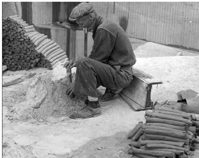
Figure 32. Filling sand bags for shooting granite.
