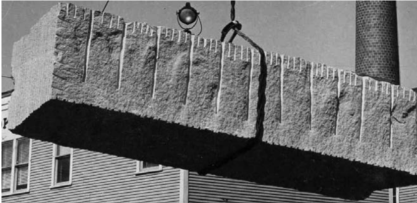
Figure 15 (above). A choke hitch.
