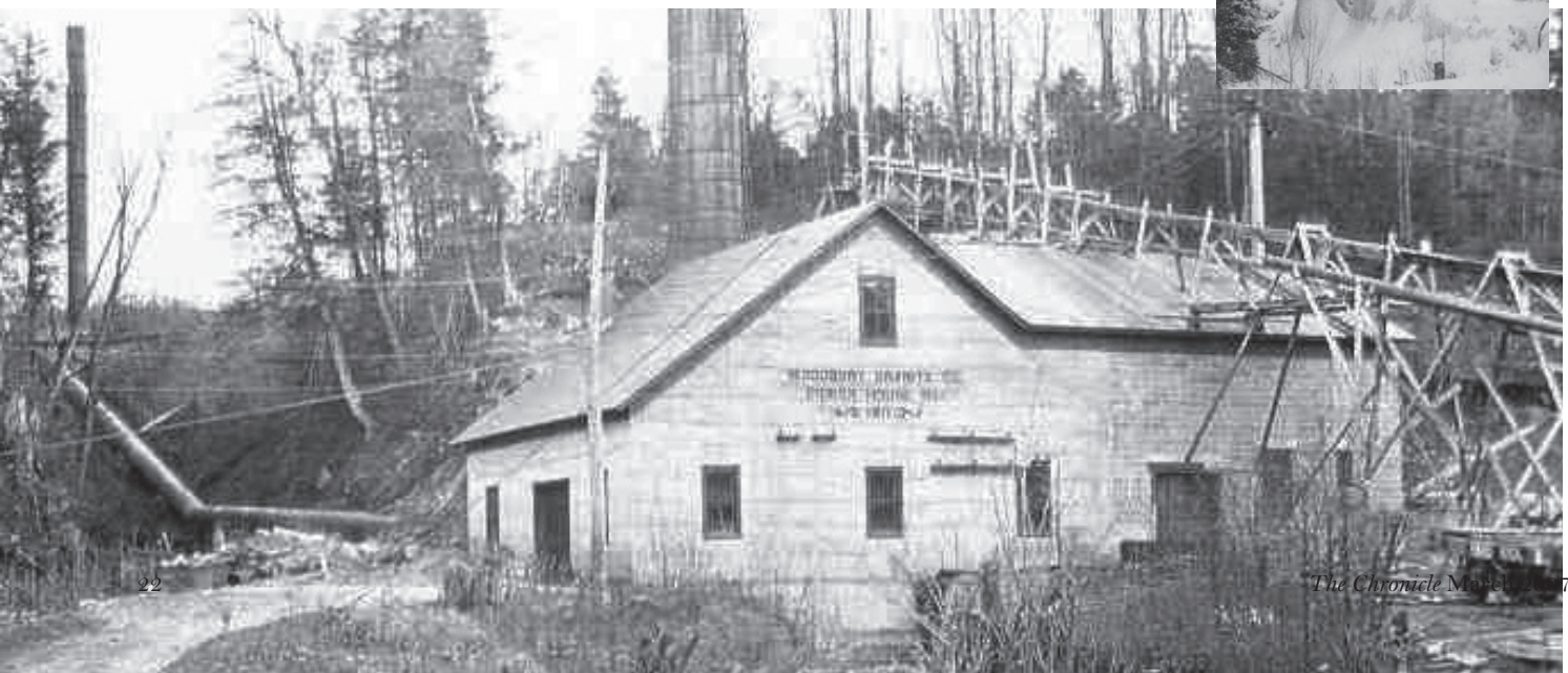
Figure 40 (right). A wintertime view of Woodbury Granite Company's power plant. The ice geysers are the result of a leaky penstock and northern Vermont's frigid winters.
