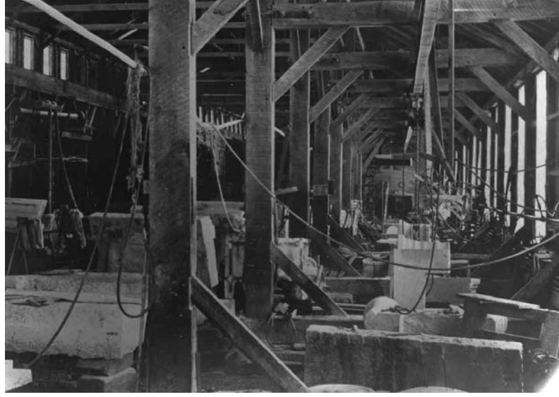
Figure 4. Straight shed side bay with a row of granite cutter and carver bankers. Note the compressed air pipe running along the right-hand wall and the hoses leading to pneumatic tools, one of which can be seen resting on a stone in the foreground.
