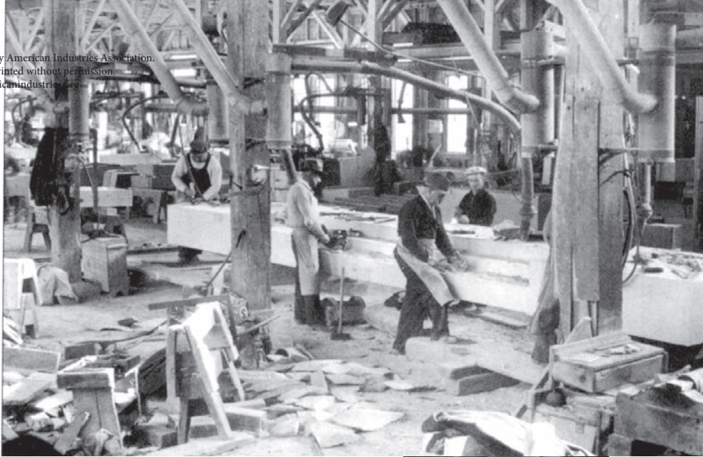
Figure 50 (above). A granite shed with an installed dust removal system. Nozzles, flexible ducts, chip traps, and rigid duct work are visible.
