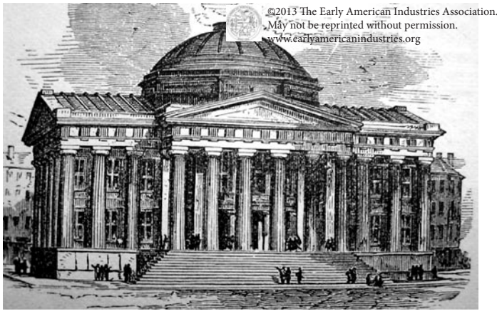
Figure 7. Boston Custom House (above). The construction of this Doric style building in the shape of a Greek cross was commenced in 1837. Thirty-two fluted columns, each weighing forty-two tons, surround the building. In 1915, a tower was added, using Cape Ann gray granite.
